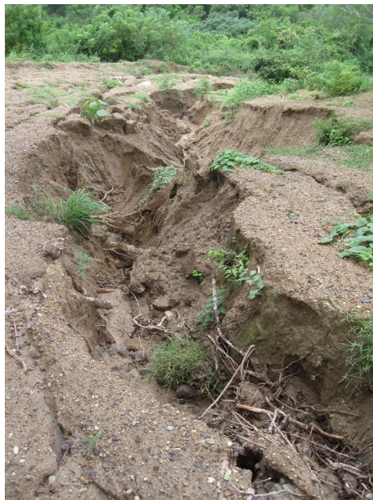
Figure 15: Gully erosion in Luriza, Usiacuri, Colombia (own picture by H. Schubert 2016)
